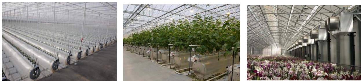
Fig. Examples of air distribution via sleeves or (on right) free outflow Source: left KUBO, right Certhon
