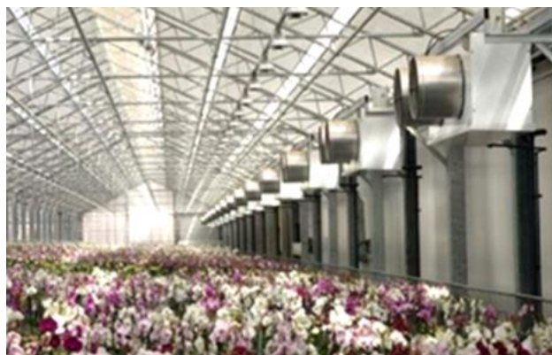
Treated air is pumped through sleeves that are under the plants, or is released above the plants.
