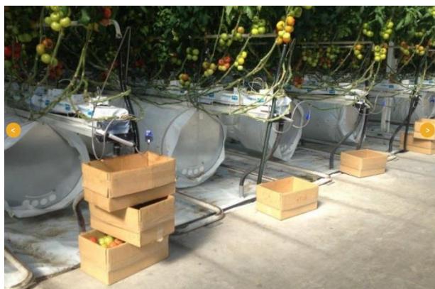
Fig. The air distribution sleeves in the Ultra-Clima greenhouse from KUBO, at D’Vine Ripe in South Australia.
