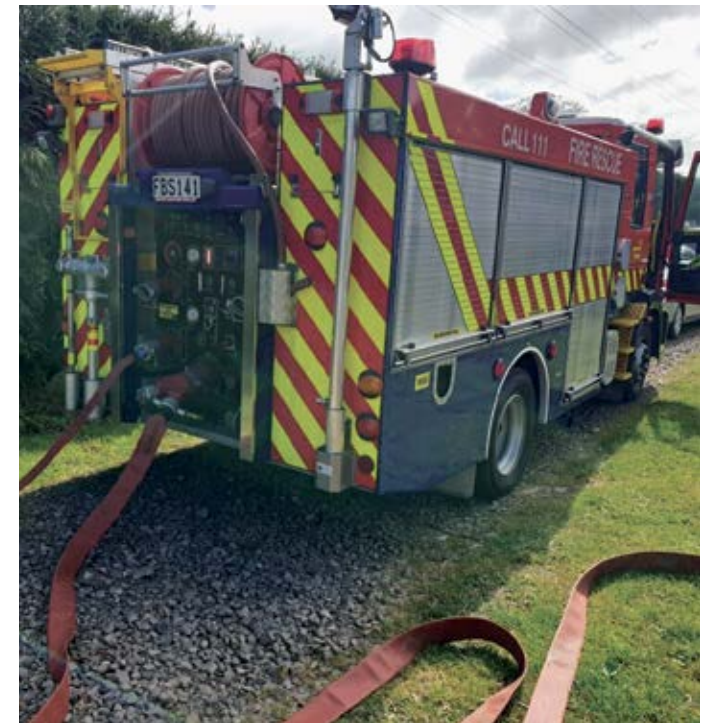
The adaptor fitted to the bore servicing two Ongare Point orchards is compatible with the equipment used by emergency services
