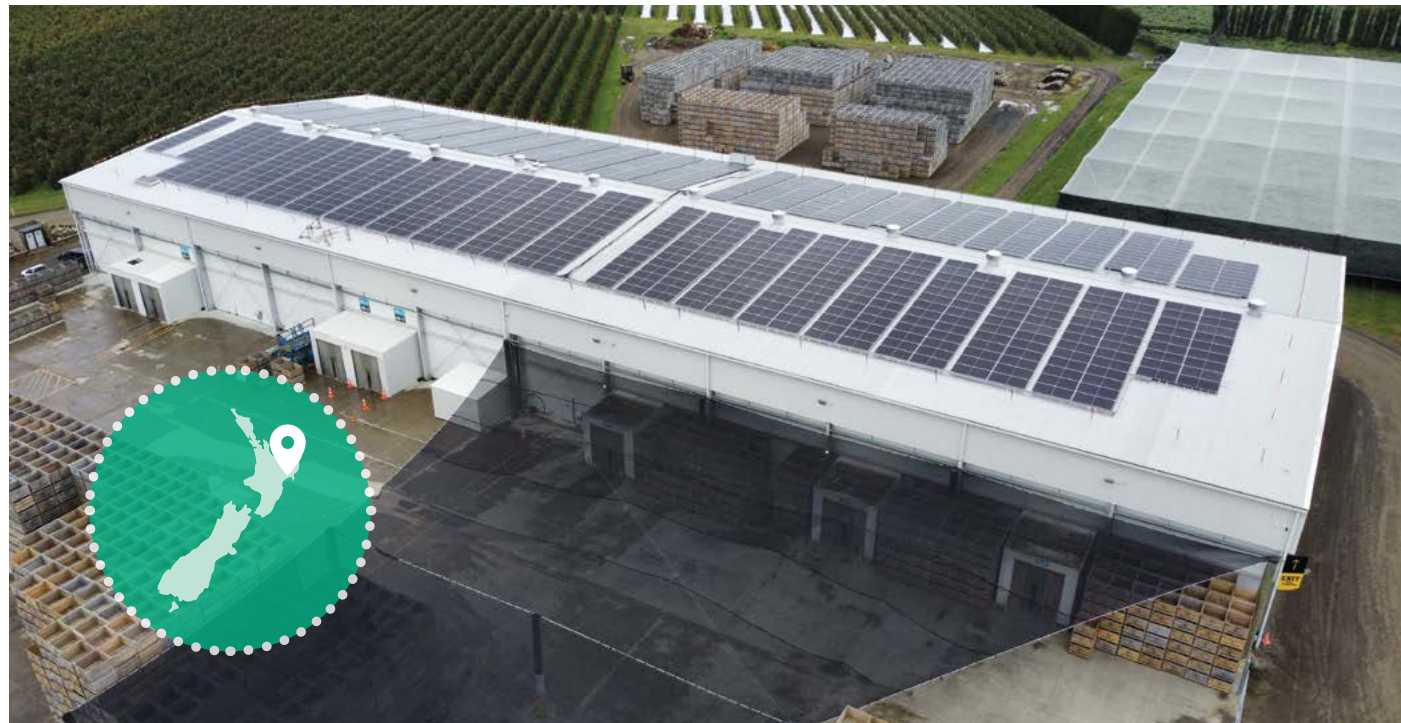
The solar panel system at Kaiaponi is likely the largest on-roof solar installation in Tairāwhiti Gisborne
