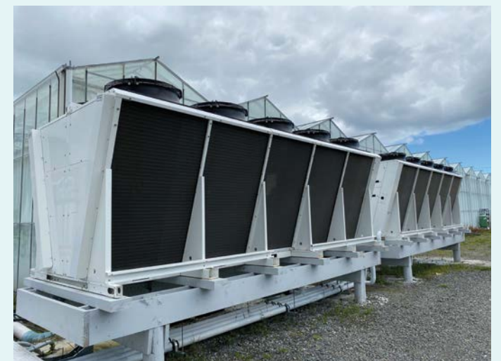
Airsides evaporators at Van Lier Nurseries
