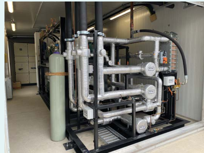
The new R744 (CO 2 ) heat pump system by Glacem Cooling Technologies
