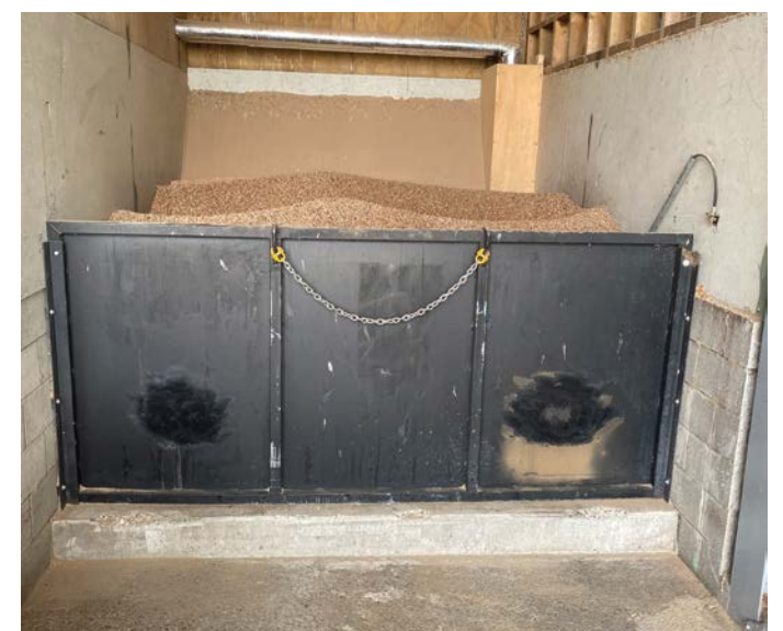
The covered area for storing the wood pellets is big enough for them to be tip loaded to drop into the feed system. Coal to wood pellet use is close to 1:1 so huge storage bunkers are not necessary
