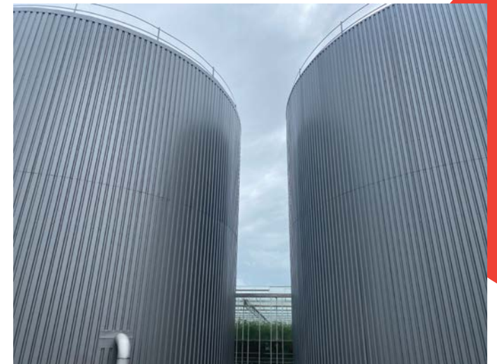
The newly installed buffer tank allows the storage of hot water with minimal heat loss
