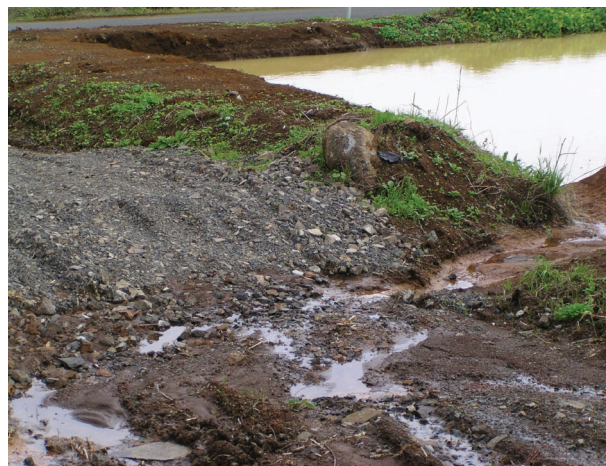
Figure 3.2: Example of a raised and metallised accessway.
