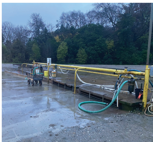
Figure 3.7: Washdown pad. Photo courtesy of Leaderbrand Gisborne.
